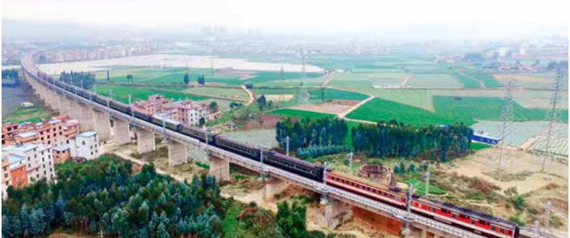
December 15, 2016: A train passes the Dalihuaying Extra-large Bridge. The bridge is located along the Kunming-Yuxi section of the China-Vietnam and China-Laos international railways. [by Zhang Xiangtao/Xinhua]
