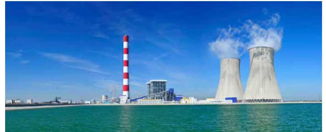
SEPCOIII has contracted India's largest foreign-funded power plant, Jhajjar Power Plant, which began operation in 2012.
